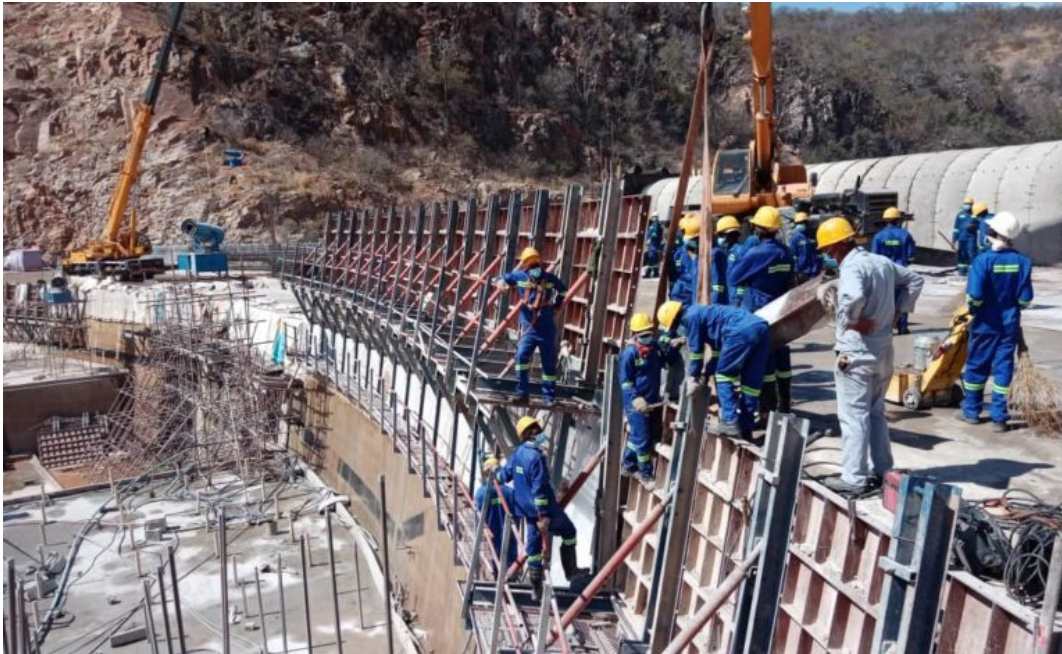
Construction of the Kunzwi Dam
