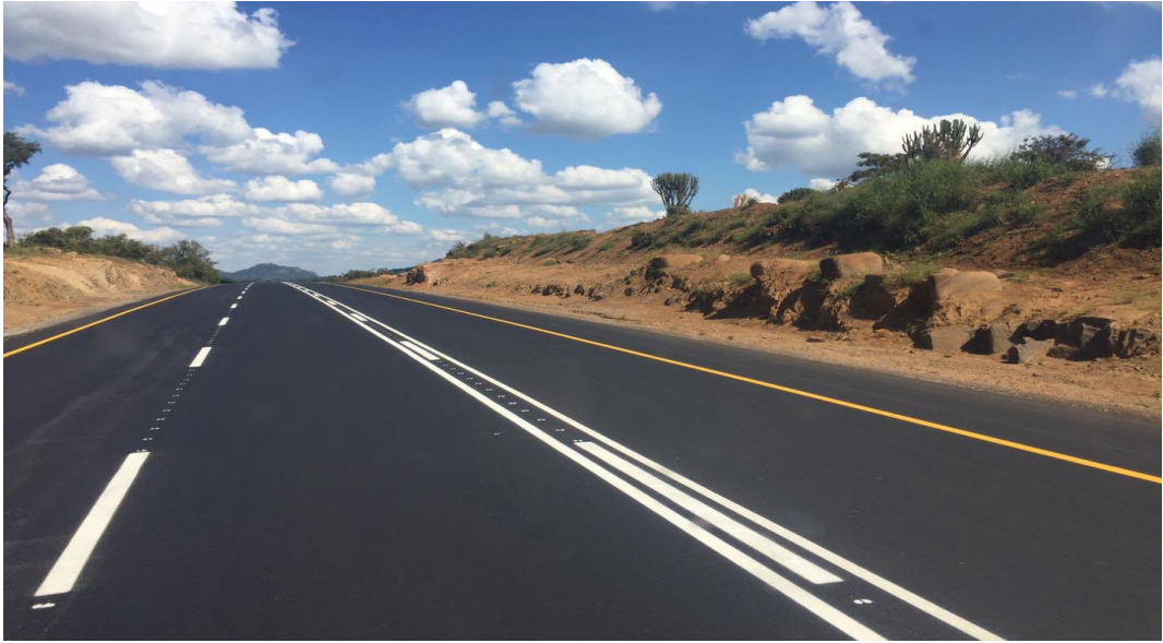
Completed section of the Harare-Masvingo-Beitbridge Highway
