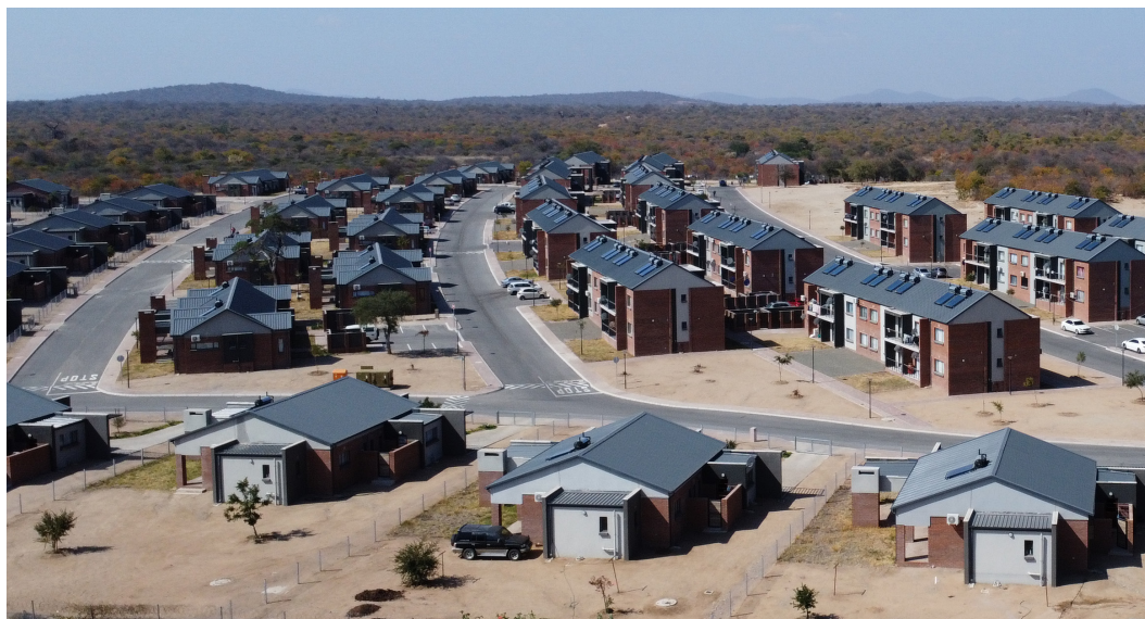
Beitbridge Border Housing. Source: Themban Media
