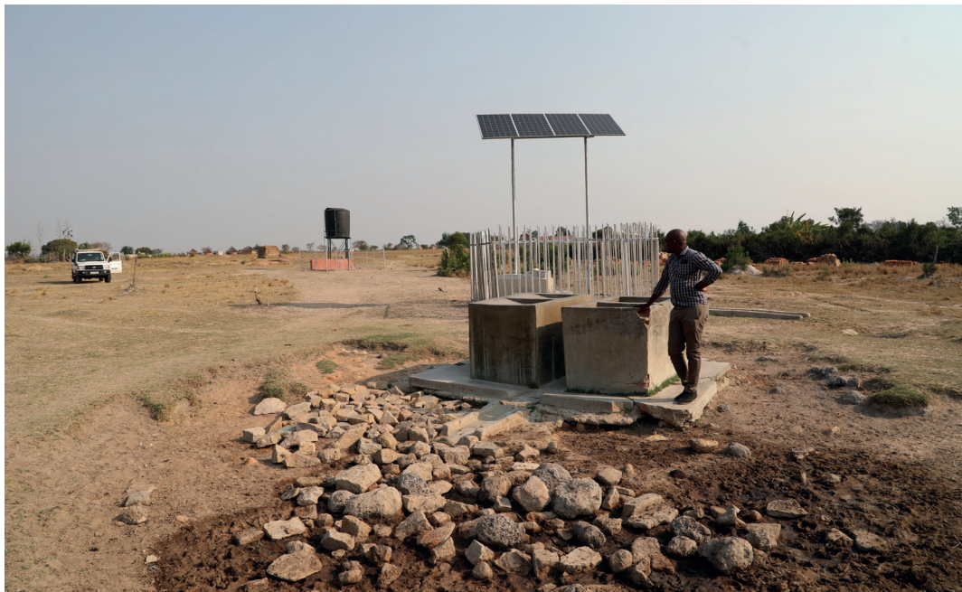
Solarised Borehole, Chikomba RDC: Themban Media
