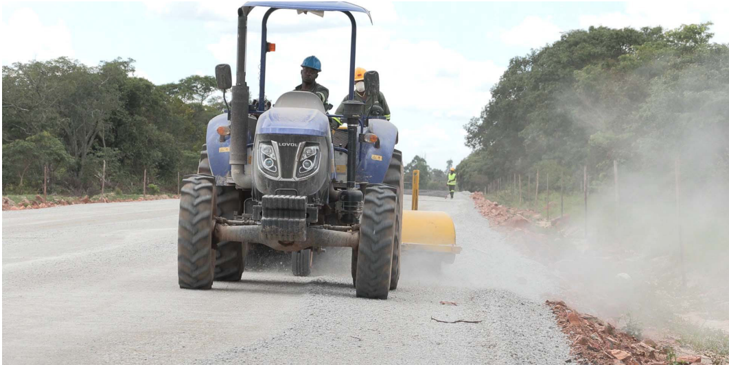
Gwanda Municipality, Jacaranda Road construction
