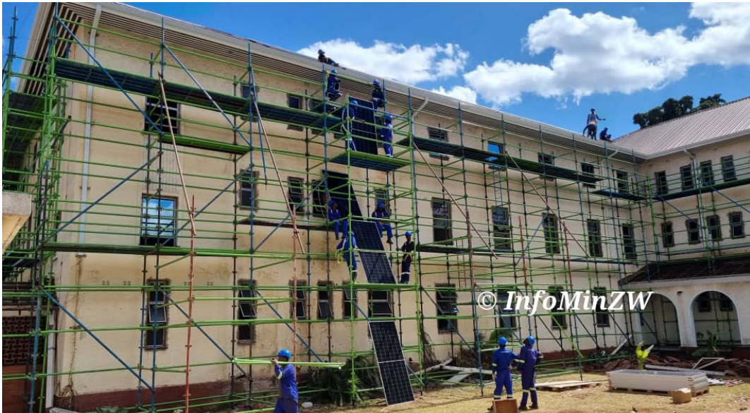
Rehabilitation of the Parirenyatwa Group of Hospitals
