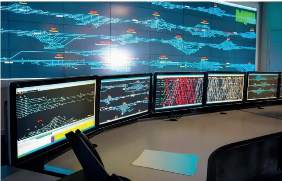
Railway Infrastructure. Source: Ministry of Transport and Infrastructural Development
