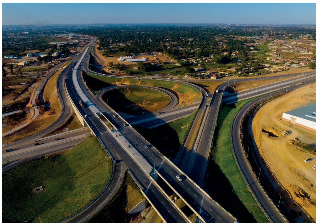
Aerial Picture of the Trabablas Interchange. Source: Them bani Media
