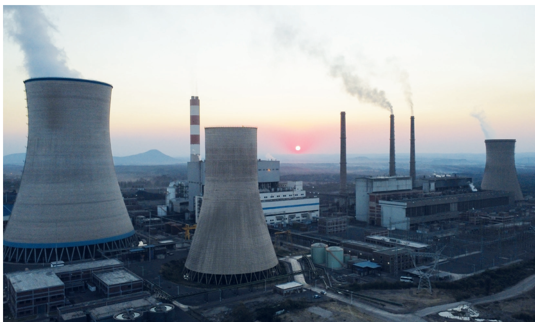
Hwange 7 & 8 Thermal Power Station. Source: Thembani Media
