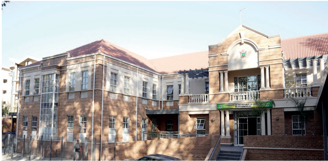
Refurbished Johannesburg Consulate
