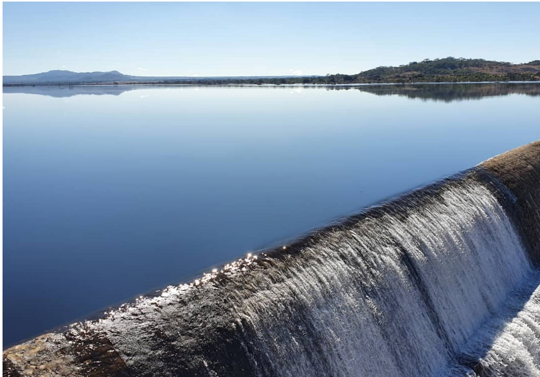
Muchekeranwa Dam in Marondera
